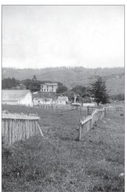
Modern reconstruction of the 1906 fence on the same site and in the same position. Note the displacement of approximately 7.6 m (25 ft) by 2006. (Photograph courtesy Tammi Grant.)
