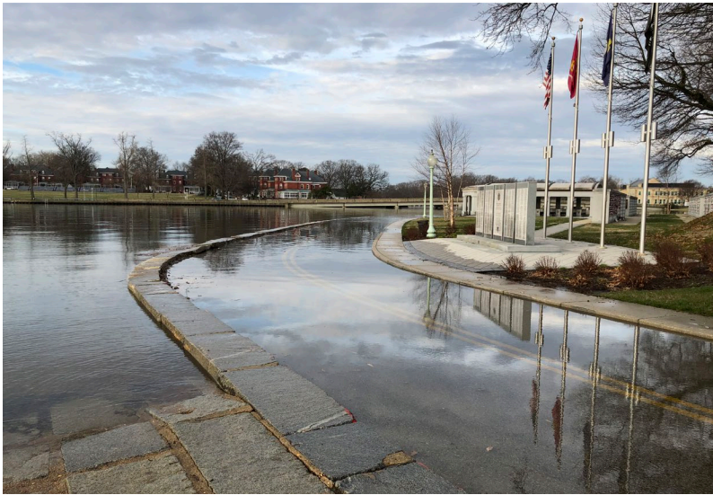
Photo 2. Ramsay Road, which runs along the cemetery on the campus of the U.S. Naval Academy, flooded more than 40 times in 2018 and 2019. Credit: David Kriebel
