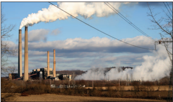
Coal-fired power plant
